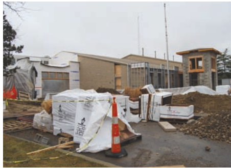
Station 91 at 6255 Shier Rings Road
