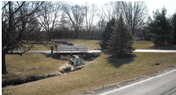
Bridges can be an access concern for the Fire Department if they are not wide or strong enough for trucks to pass.
